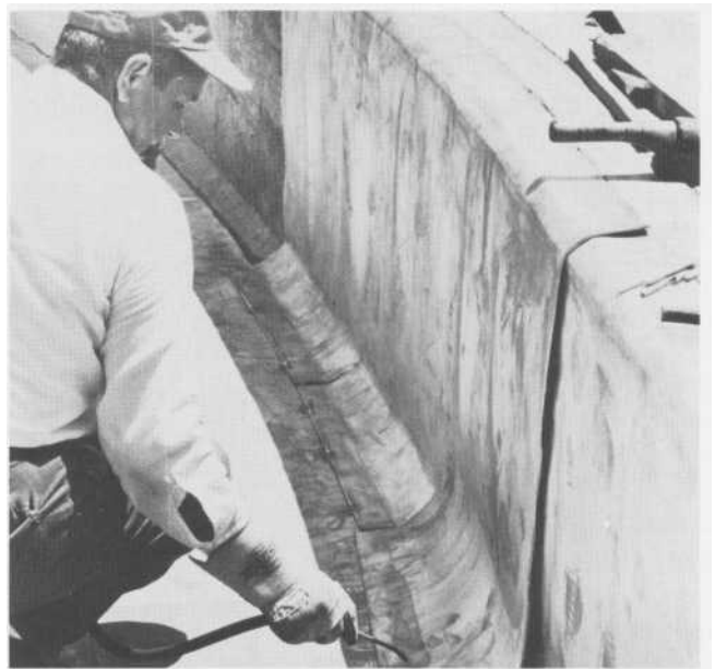
Reflecting pools and decorative fountains make extensive use of sheet lead waterproofing. The sheets on the sides are formed to follow the cant profile, then burned (welded) and flashed to other sheets to complete the waterproofing integrity.
